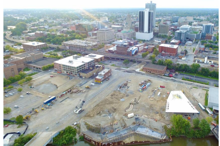
Construction of Promenade Park (right foreground), Site to left
